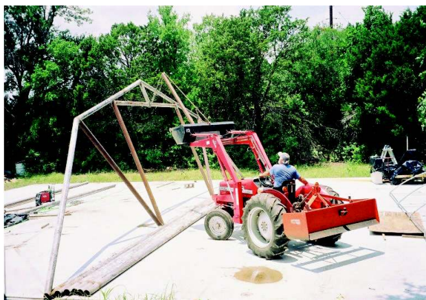
Raising the first truss
