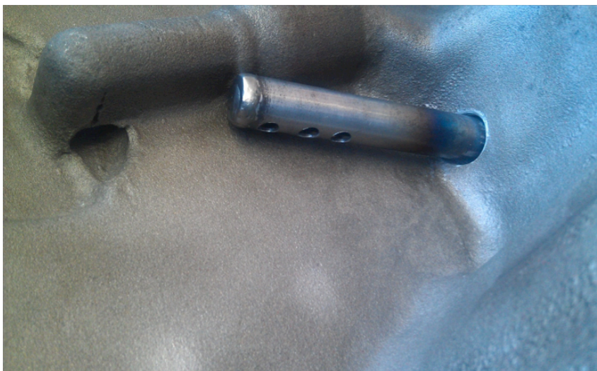
new antivortex suction tube installed
