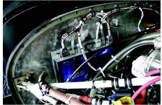
Controllers on firewall
